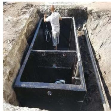
The preparations on the headworks structure at the plant for the new odor control scrubber system that is forecasted to be delivered in January 2020 began this week. The new odor control scrubber is being constructed by the City's contractor Evoqua Water Technologies. A drainage pipe had to be installed for the scrubber's operations as one of the requirements.
