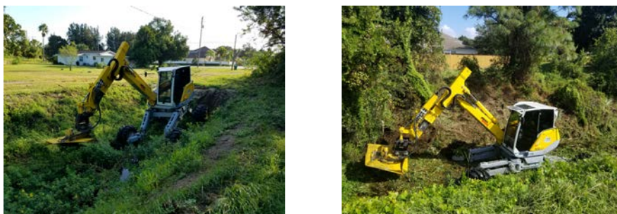
Images of canal maintenance.
