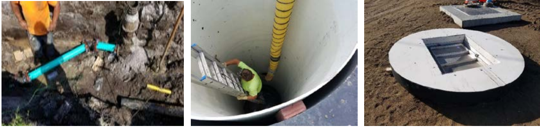
Images of wet well u-lining.
