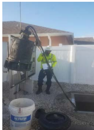
Images of lift station pump being serviced.
