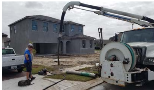
Image of sewer blockage being removed.
