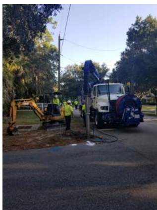
Images of Vac-Con truck assisting with locates.
