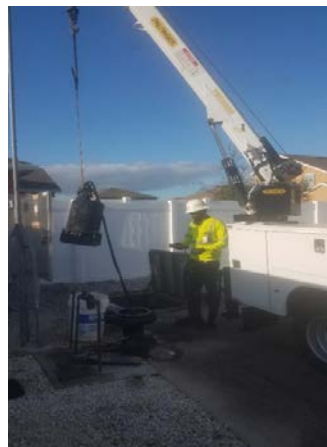
Images of lift station pump being serviced.
