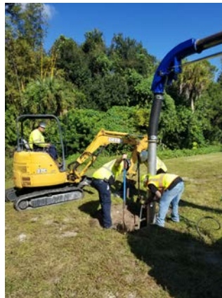
Images of Vac-Con truck assisting with locates.
