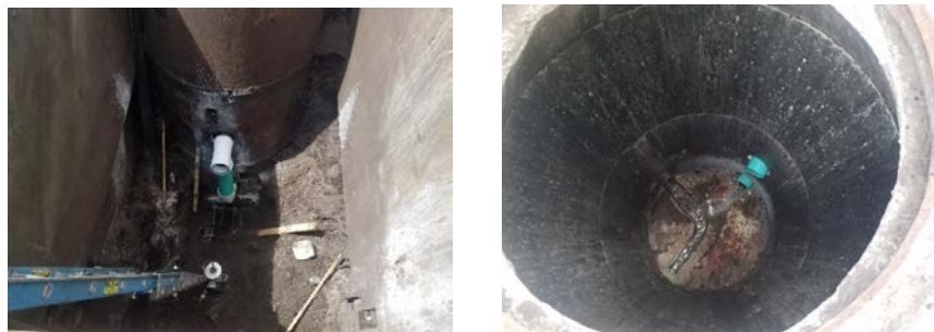
Images of Havens lift station inspection.
