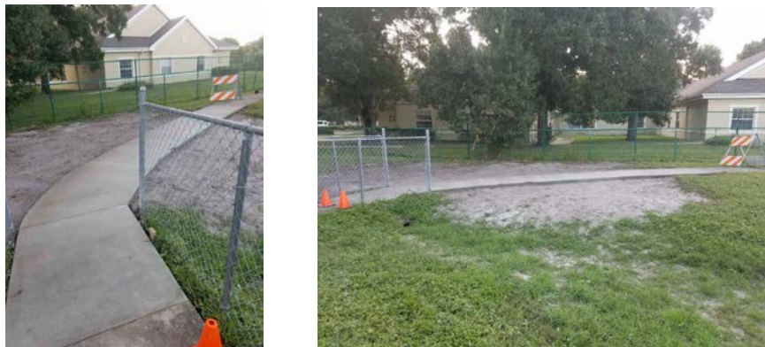
Images of sidewalk repair on Greenboro Drive.
