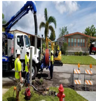
Images of service line installation in Hollywood Estates.
