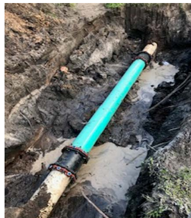
Images of force main break repair.
