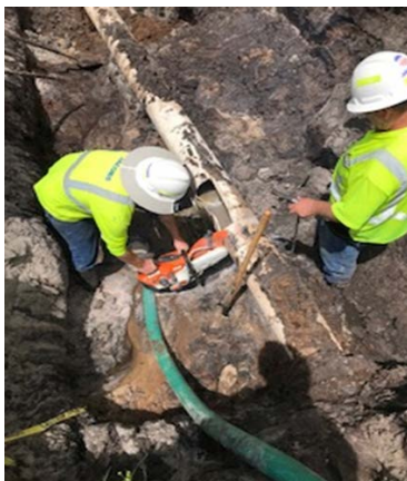
Images of force main break repair.
