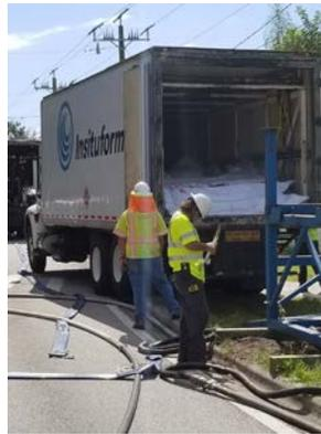
Images of contractor lining drainage pipes.
