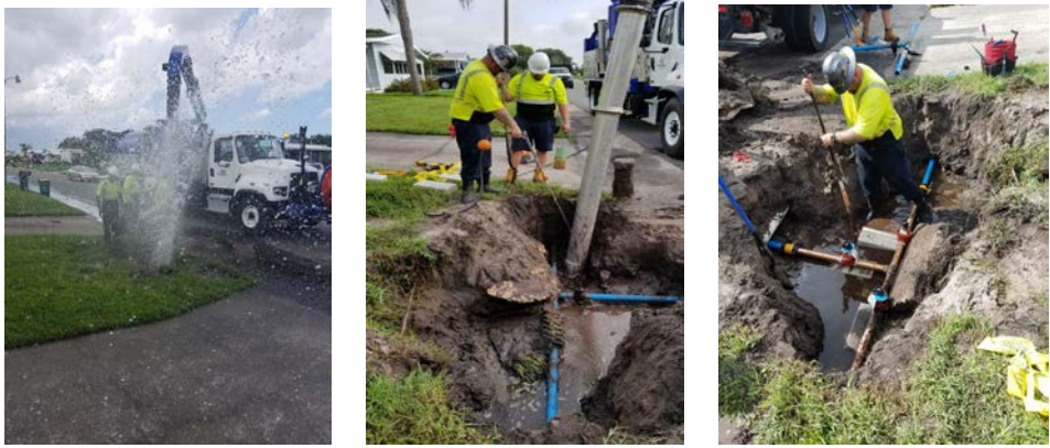
Images of City employees repairing a water main.
