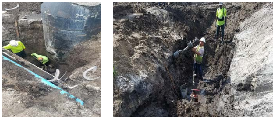
Images of construction site inspections.
