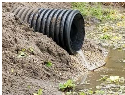
Images of new stormwater drainage pipe at Buena Vida.
