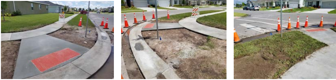
Images of sidewalk and curbing on Potenza Drive.
