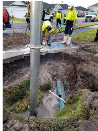
Images of employees repairing water main break on Potenza Drive.
