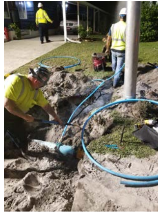
Images of employees repairing water main break on Boone Avenue.
