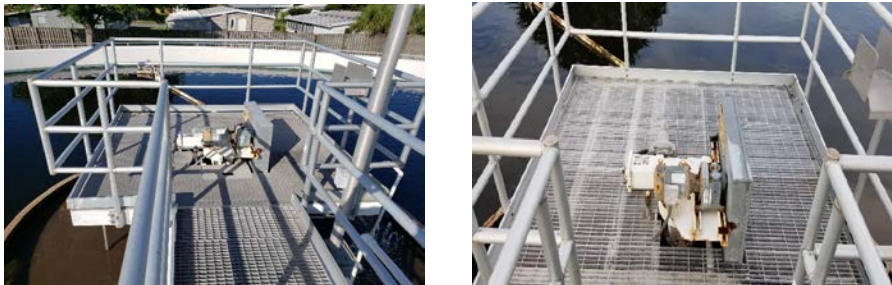
Images of new open floor grating on clarifier.
