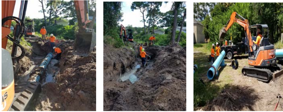
Images of contractor repairing water main.
