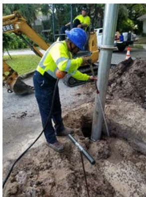
Images of City employee repairing a service line leak.
