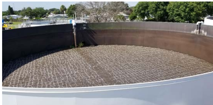
Image of aeration basin at sewer plant.
