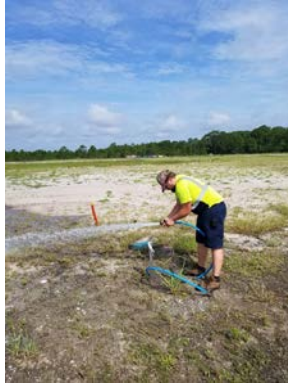
Image of City employee repairing water service leak.
