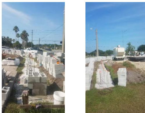
Images of VMC lift station and wall construction.
