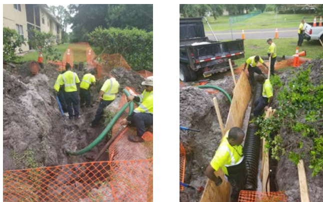
Images of City employees working on drainage pipe.
