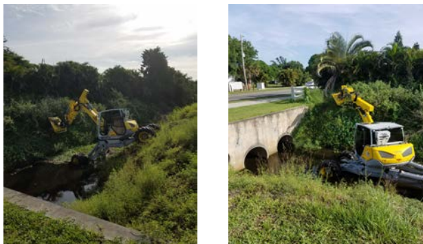
Images of Menzi Muck cleaning C1-E canal.
