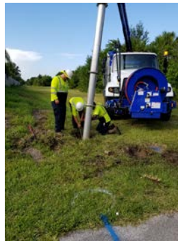
Image of City employees verifying pipe location.
