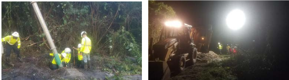
Images of Jacobs employees repairing force main.
