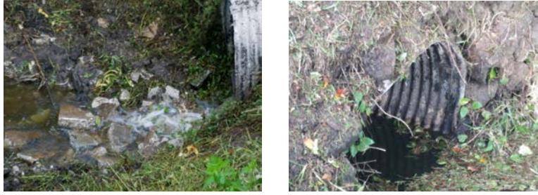
Images of intake and outfall of storm drain pipes.
