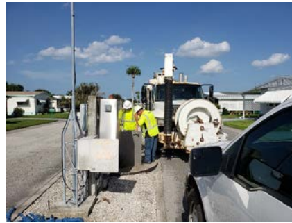
Images of Jacobs employees removing blockage from manhole on Gail Boulevard.
