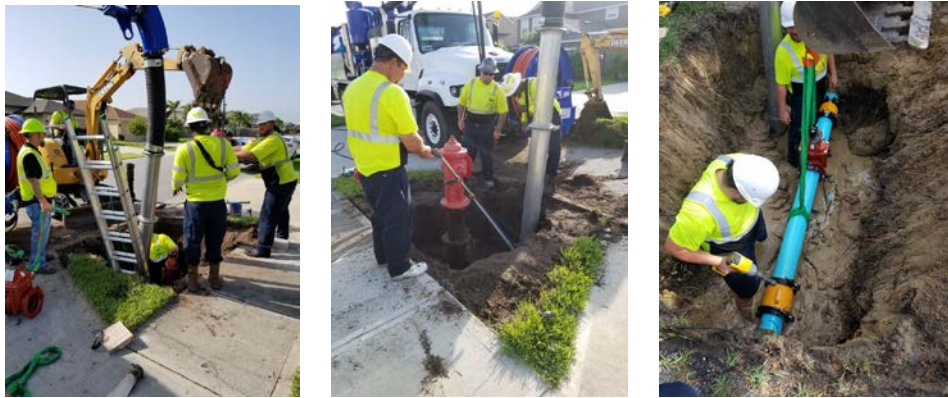
Images of City employees replacing valves.
