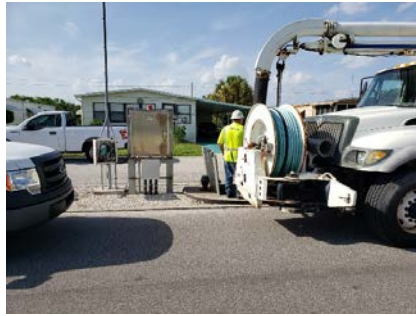
Images of Jacobs employees removing blockage from manhole on Gail Boulevard.
