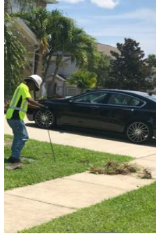
Image of Jacobs employee testing backflow device in Hammock Lakes East.
