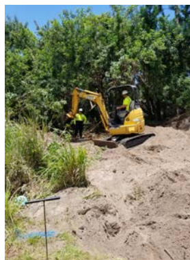
Image of City employee training on mini excavator.
