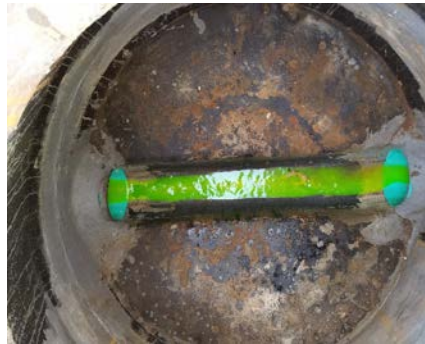
Images of gravity sewer in parking lot and green dye testing.
