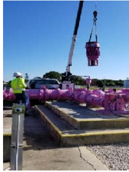
Image of transfer pump installation at sewer plant.
