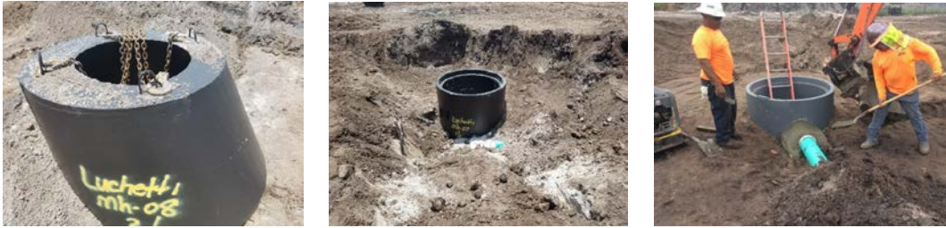
Images of new manhole installations at Springs of Hibiscus apartments.
