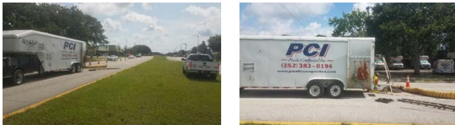
Images of PCI repairing manhole on U.S. 192.
