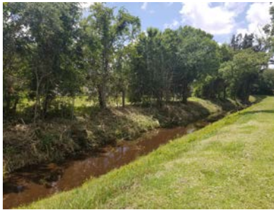
Image of C-3 canal in Clements Wood neighborhood.
