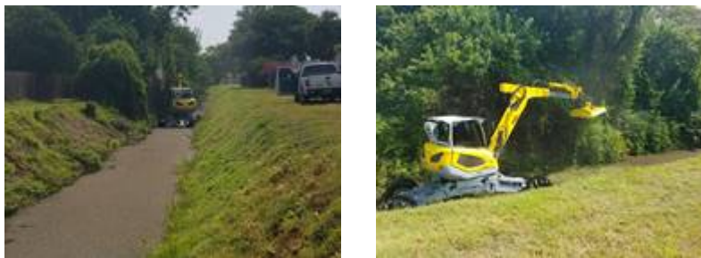
Images of the Menzi Muck cleaning the C-6 canal in Clements Woods.
