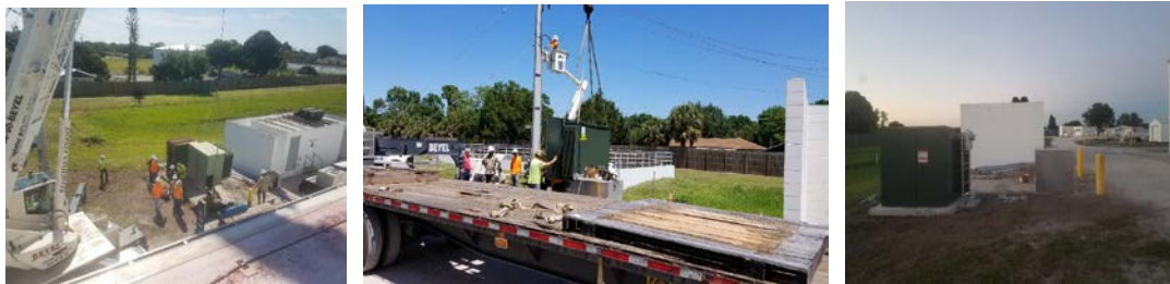
Images of FP&L installing switch and transformer at sewer plant.
