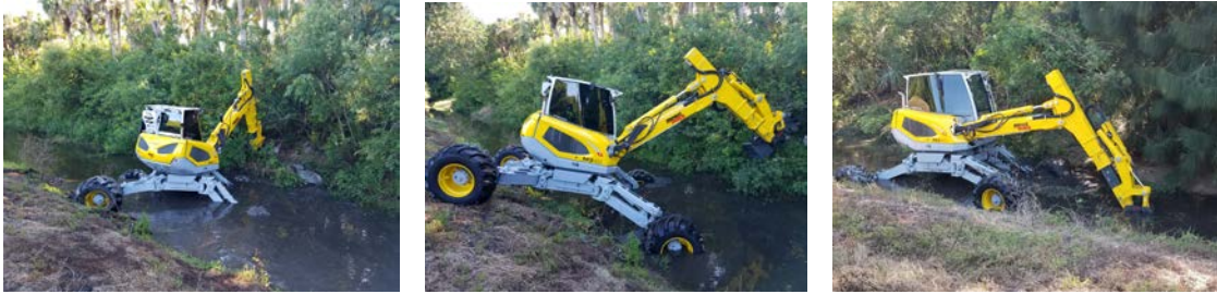
Images of Menzi Muck cleaning canal on Coastal Lane.
