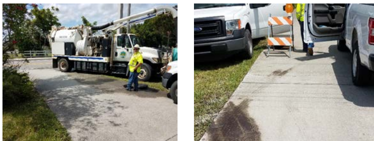
Images of employees removing sewer blockage in Hollywood Estates.
