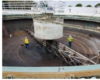
Images of rake arms on clarifier at sewer plant.
