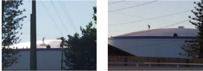
Images of ground storage tank at plant.
