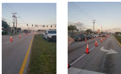
Images of Maintenance of Traffic pattern to assist workers.
