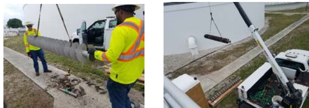
Images of grit cyclone augur/screw installation at sewer plant.
