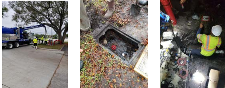
Images of water line repair on W. New Haven Avenue.
