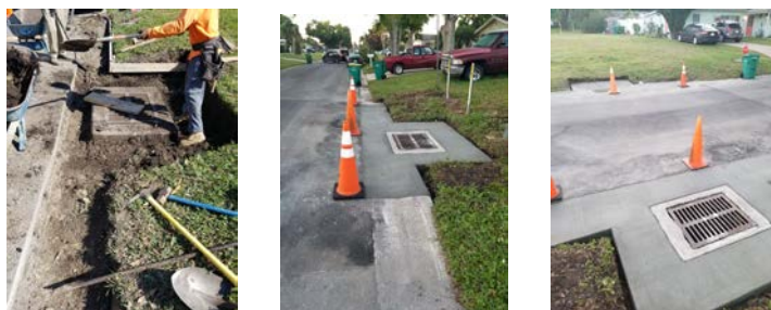
Images of new curbing installation on Monaco Road.
