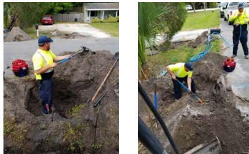
Images of water line installation on Shannon Avenue.
