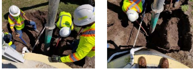
Images of crew repairing a reuse pipe leak at the plant.
